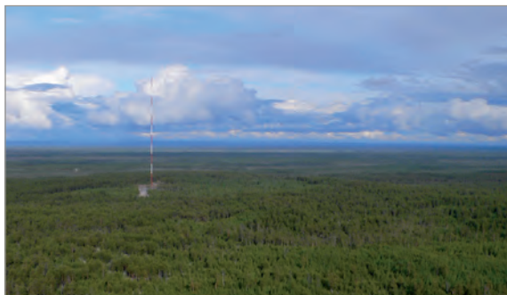
Zotino Tall Tower Observatory: a 300 m tall mast for the long-term monitoring of biogeochemical trace gases, aerosols and atmospheric chemistry established in central Siberia by the MPI for Biogeochemistry, the MPI for Chemistry and the Institute of Forest, Krasnojarsk; funded by the Max-Planck-Society.
