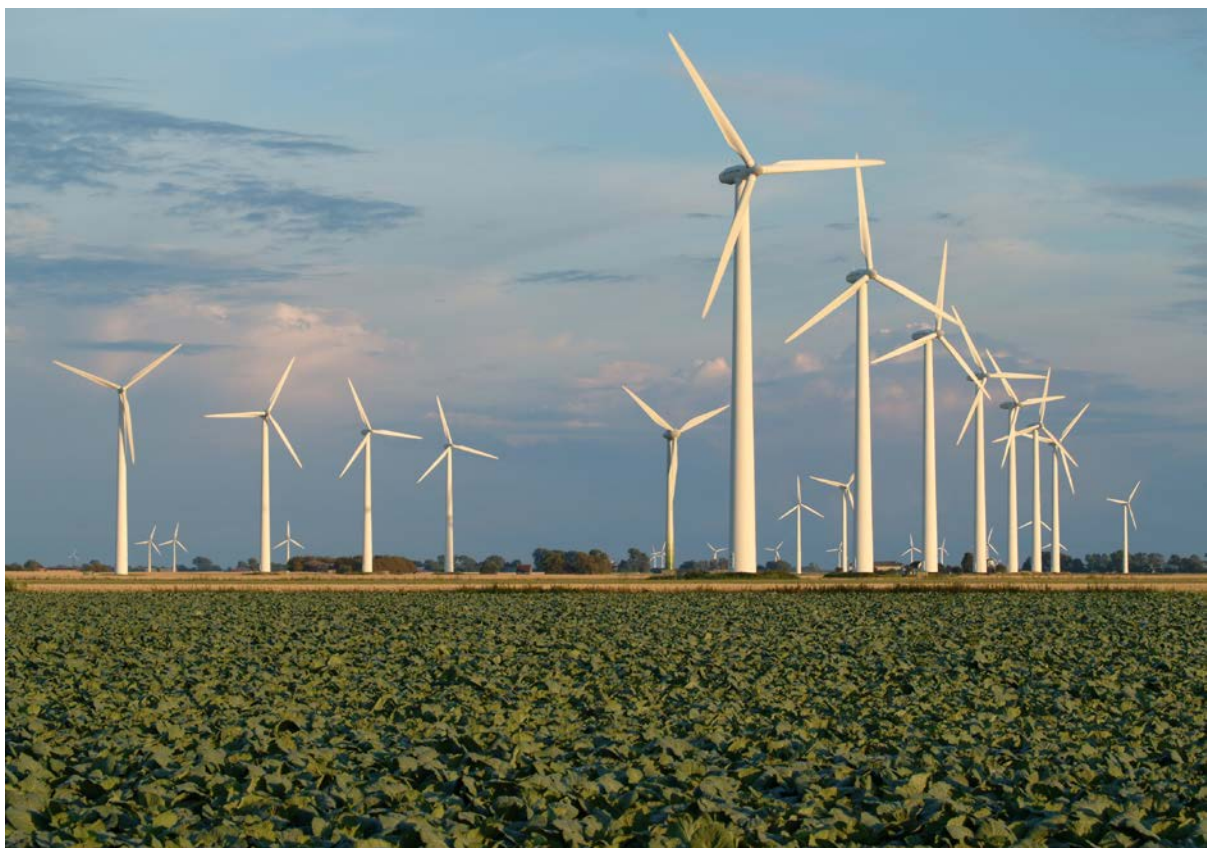
Small wind farm with several turbines
